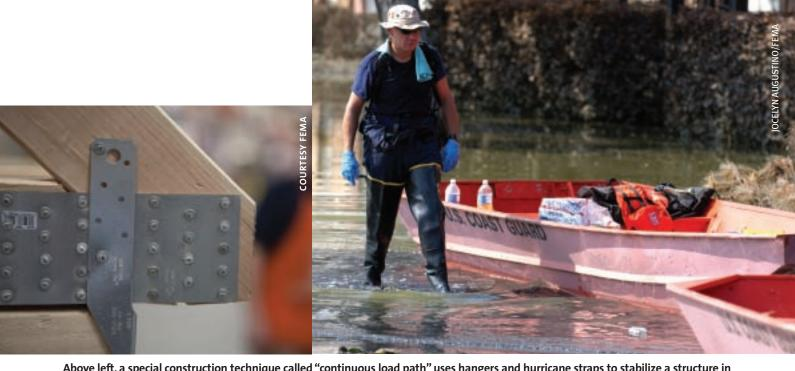
Above left, a special construction technique called "continuous load path" uses hangers and hurricane straps to stabilize a structure in severe weather, like that caused by Hurricane Katrina, which brought members of the U.S. Coast Guard out into the flooded streets for search and rescue operations.
